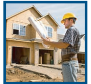
On the job site
